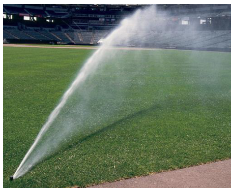
Figure 9 stationary sprinkler irrigation (mnrainman, 2015)
